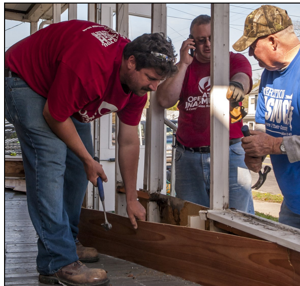
One of the many restoration projects completed during Operation Inasmuch 2015.
